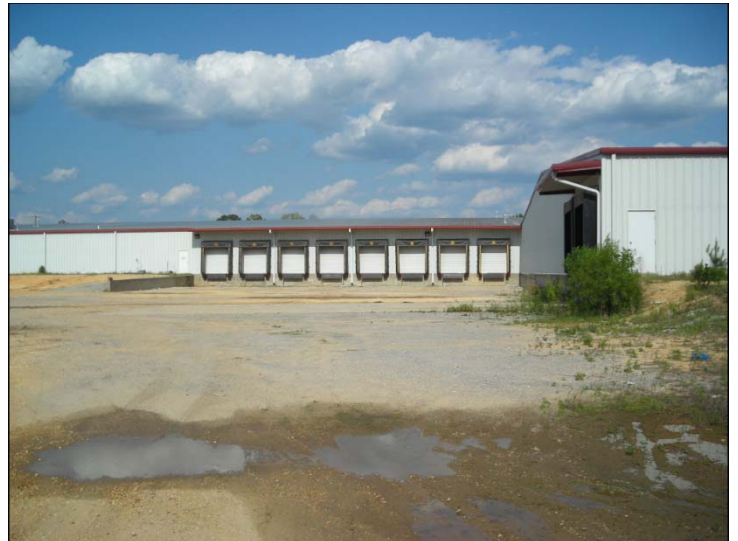
West side of building with 8 of the dock doors
