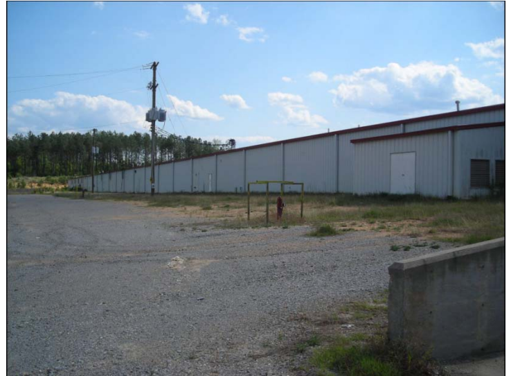
East side of building
